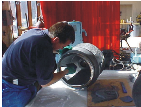
CeramAlloy CP + AC was used to smooth out and rebuild eroded areas of both impellers.
