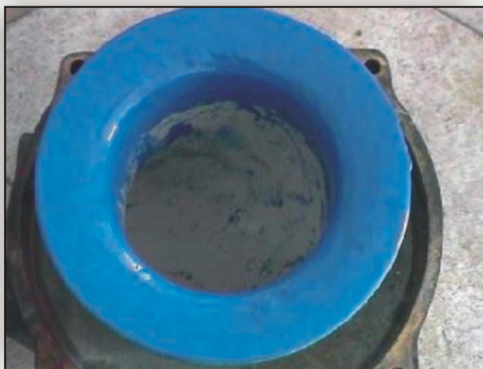
DuraTough DP applied to re-build damaged surface.
