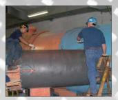
METALCLAD® DuraWrap® can be applied to the interior and / or exterior of piping and equipment to both seal and strengthen these components. When applied to the interior walls of underground or otherwise inaccessible piping, METALCLAD® DuraWrap® can effectively repair and restore piping integrity without expensive excavation and replacement.
