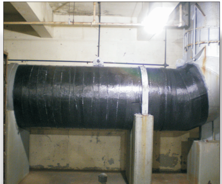
Completed DuraWrap System.
