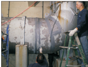
After grit blasting, leaks repaired with DurAlloy.
