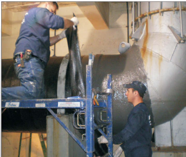
DuraWrap Carbon Fiber, impregnated with DuraWrap Polymers, being wrapped around pipe section.
