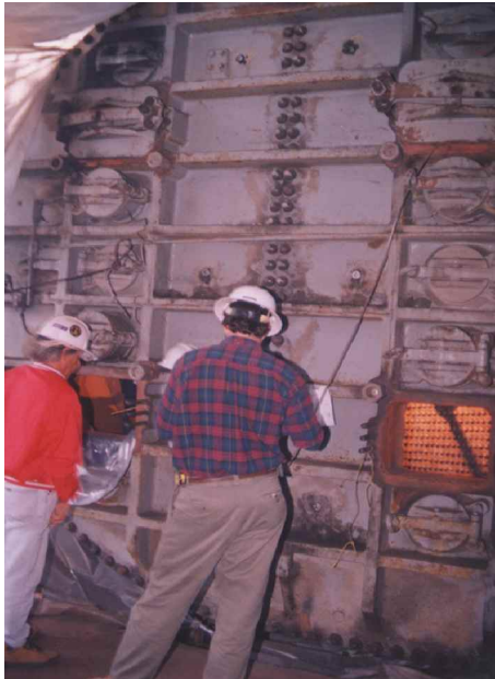
Engineers inspect one of the massive waterboxes at the power station.
