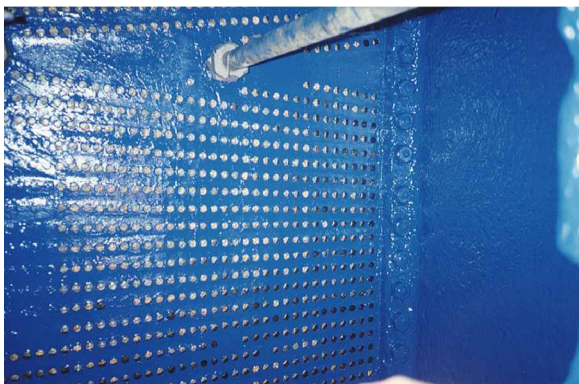
Final coat of CeramAlloy CL+ (Blue) applied to all wet surfaces to provide years of erosion/corrosion protection to the condensers.
