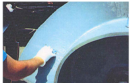
Rebuilding with CeramAlloy CP+
