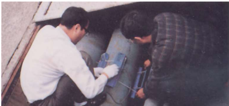
Four pair of ENEFLOW 5000 Fluid Dynamic Power Cells being installed on one of the main ash slurry lines.
