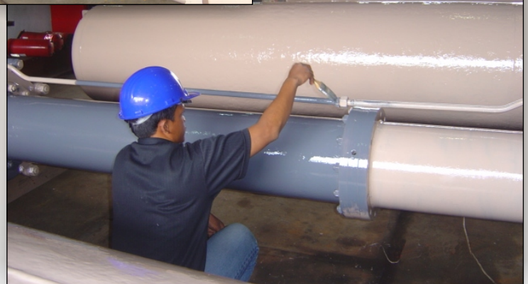
Final coat of CHEMCLAD SC being applied.
