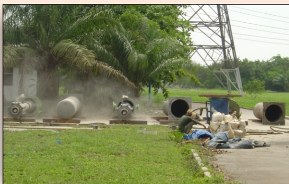
All pump sections were grit blasted.
