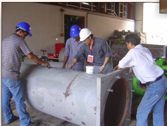
DurAlloy being applied to repair pitted areas.
