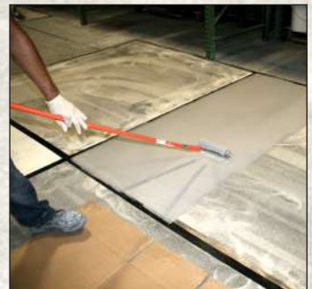
SuperBond ™ is a surface tolerant primer with an extended overcoating window.
